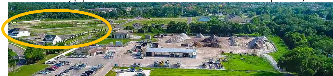
Stormwater Maintenance Yard
